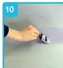
Apply 2-3 coats of OTL 025 Tanking Compound
