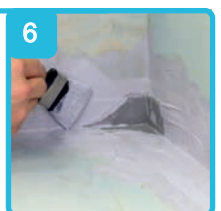
Applying OTL 028 (Internal Corner) or OTL 029 (External Corner)
