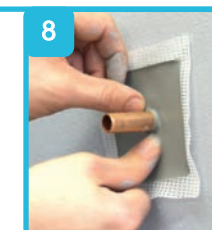
Applying OTL 026 Pipe Sleeve
