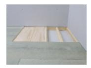
5. Full sized OTL waste support is used to build a false floor between the joists using 25mm x 50mm softwood battens secured to the side of each of the joists with 50mm No.8 Countersunk woodscrews @ 150mm centres. Position the top of the battens 24mm below the top of the joists ready to recieve 24mm OTL waste support. Cut the OTL waste support to fit between the joists.
