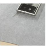
**12.** Place the former over the channel and cut the exposed tanking mat and remove this piece. (3-5mm of metal on the frame should be left exposed).
