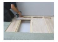
With the waste support in place, with a pencil mark the position of the channel on joists, remove the false floor panels and where the pencil marks are on the joists notch to a depth of 25mm to allow for the channel. Cut 400mm off the panel where the waste outlet is situated and set the other piece aside. Secure all the false floor panels (except for the piece set aside) to the joists and battens.
