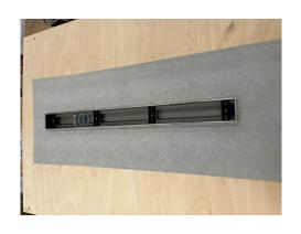
11. Remove the roll of tanking mat and lay over the drain. Peel the backing tape from one corner then back 150mm. Apply enough pressure for the mat to adhere to the tray. Lifting up the tanking mat gently remove the backing tape 300mm at a time, apply pressure to the mat and stick down.
