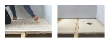
4. Place the former in position and mark out the hole on the waste support for the waste outlet, remove the former and waste support and cut out the hole in the 24mm plywood for the waste outlet.
