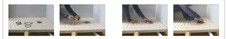
9. Ensuring the large thick rubber washer is on top of the lower part of the gully body, place the stainless steel plate (with the countersunk holes to the top) into position on the former. Place the top rubber waste seal over the flange, screw the flange through the stainless steel plate into the lower part of the gully body. Leave hand tight.
