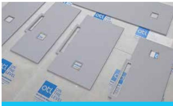
Because the formers were large (in one case 2.6m x 1.1m) OTL decided to increase the gradient from the norm, thus providing much better water flow to the gully. In the extremely unlikely case of any water flowing away from the gully this was simply an added precaution.
