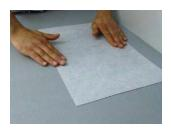
Place the Butyl tanking mat centrally over the drain. Peel back 75mm of the backing tape from one end and gently press down into position on the former. Slowly working towards the other end, pull the backing tape from the tanking mat, pressing down firmly from the middle out until the tape is in position. With the backing tape removed and the tape in position, press down firmly.
