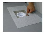
Push the centre of the mat into the edges of the drain. With a sharp knife cut out and remove the excess mat over the drain. Push the edges of the tanking mat firmly into the drain.
