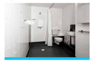
On The Level supplied 60 custom level access formers measuring 1200mm x 1200mm for this project. All formers have a central waste and standard gully and were designed for level access wet rooms installed in accessible bathrooms with vinyl sheet flooring.
