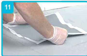
Place the tanking mat over the gully with the hole positioned centrally. Fold one side of the mat over and apply a coat of compound, bed down the mat and repeat to the other side
