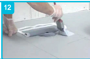
Place the tanking mat over the gully with the hole positioned centrally. Fold one side of the mat over and apply a coat of compound, bed down the mat and repeat to the other side
