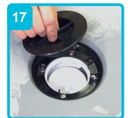
Insert the trap protector. Replace the coverplate on completion
