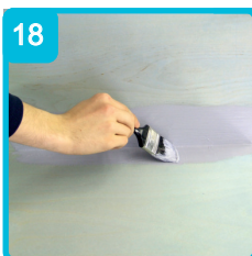
Apply 2-3 coats of OTL 025 Tanking Compound
