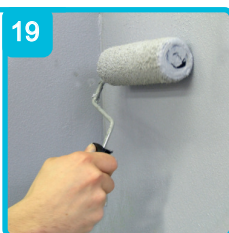
Apply 2-3 coats of OTL 025 Tanking Compound
