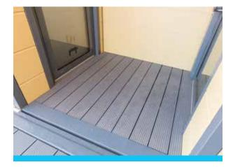
We were also delighted to adapt our product once again and assist with providing a terrace floor. Taking the principle of an internal wet room and placing it in an external environment by introducing gradients into the terrace surface, keeping water under control and forcing the water to the outlet. The terrace was to be covered with a metal grating, however our innovative Exterior Tanking kit was used to ensure the terrace remains watertight, and water only escapes via the outlet.
