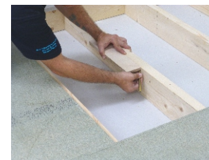
5. Build a false floor between the joists using 25mm x 50mm softwood battens secured to the side of each joists with 50mm No 8 countersunk woodscrews @ 150mm centres. Position the top of the battens 18mm below the top of the joists ready to receive 18mm WPB Plywood. Cut pieces of 18mm WPB plywood (NOT SUPPLIED) to fit between the joists.
