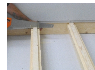
7. With the shoulder removed place the former in position, with a pencil, mark the position of the channel on the false floor, remove the former and false floor panels and cut out for the channel, where the pencil marks are on the joists notch out the joists to a depth of 20mm to allow for the channel. Cut 400mm off the panel where the waste outlet is situated and set the other piece aside. Secure all the false floor panels (except for the piece set aside) to the joists and battens.
