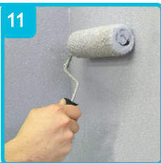
Apply 2-3 coats of OTL 025 Tanking Compound
