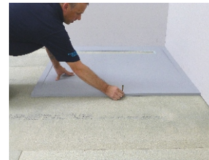
1. Place the former on the floor. With a pencil mark its position on the floor
