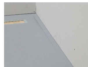
6. With the plywood in position place the former in position and butt up against the wall, with a pencil mark the finishing line of the plaster. Remove the former, measure the depth of the plaster line (A), mark the depth of the plaster line on the other side of the shoulder, draw a line and cut off the excess material so the fall on the former fits under the plaster
