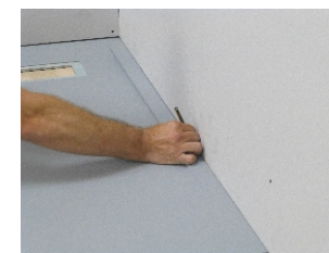
6. With the plywood in position place the former in position and butt up against the wall, with a pencil mark the finishing line of the plaster. Remove the former, measure the depth of the plaster line (A), mark the depth of the plaster line on the other side of the shoulder, draw a line and cut off the excess material so the fall on the former fits under the plaster
