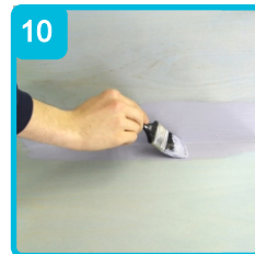
Apply 2-3 coats of OTL 025 Tanking Compound
