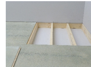
3. If the edge of the former does not rest on the joist remove the flooring back to the next joists.
