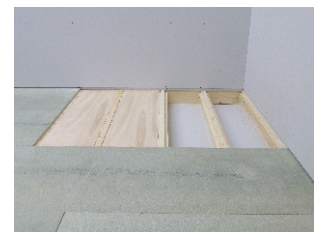
5. Build a false floor between the joists using 25mm x 50mm softwood battens secured to the side of each joists with 50mm No 8 countersunk woodscrews @ 150mm centres. Position the top of the battens 18mm below the top of the joists ready to receive 18mm WPB Plywood. Cut pieces of 18mm WPB plywood (NOT SUPPLIED) to fit between the joists.
