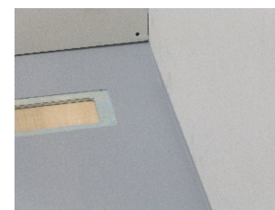
7. With the shoulder removed place the former in position, with a pencil, mark the position of the channel on the false floor, remove the former and false floor panels and cut out for the channel, where the pencil marks are on the joists notch out the joists to a depth of 20mm to allow for the channel. Cut 400mm off the panel where the waste outlet is situated and set the other piece aside. Secure all the false floor panels (except for the piece set aside) to the joists and battens.
