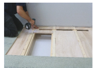
7. With the shoulder removed place the former in position, with a pencil, mark the position of the channel on the false floor, remove the former and false floor panels and cut out for the channel, where the pencil marks are on the joists notch out the joists to a depth of 20mm to allow for the channel. Cut 400mm off the panel where the waste outlet is situated and set the other piece aside. Secure all the false floor panels (except for the piece set aside) to the joists and battens.
