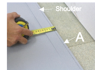
6. With the plywood in position place the former in position and butt up against the wall, with a pencil mark the finishing line of the plaster. Remove the former, measure the depth of the plaster line (A), mark the depth of the plaster line on the other side of the shoulder, draw a line and cut off the excess material so the fall on the former fits under the plaster
