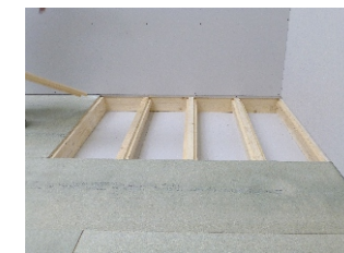
5. Build a false floor between the joists using 25mm x 50mm softwood battens secured to the side of each joists with 50mm No 8 countersunk woodscrews @ 150mm centres. Position the top of the battens 18mm below the top of the joists ready to receive 18mm WPB Plywood. Cut pieces of 18mm WPB plywood (NOT SUPPLIED) to fit between the joists.
