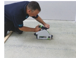
2. Remove the former and cut out the floor.
