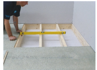
4. With the flooring removed check the joists are level.
