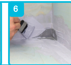
Applying OTL 028 (Internal Corner) or OTL 029 (External Corner)
