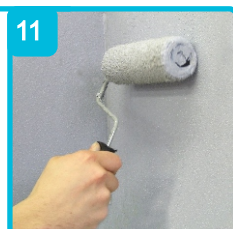
Apply 2-3 coats of OTL 025 Tanking Compound
