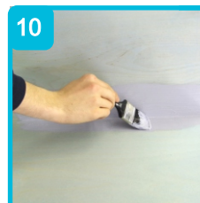
Apply 2-3 coats of OTL 025 Tanking Compound
