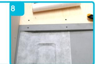
Lift up the tanking mat and gently removing the backing tape approx 300mm at a time, apply pressure to the mat and stick down. Fold the mat into the tray the other end and trim with a sharp knife.
