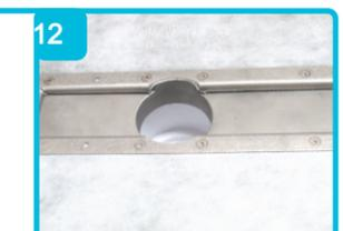
Position the clamping ring into the main channel and push down. Screw the clamping ring to the main channel through the tanking mat. With a sharp knife cut along the inside of the clamping ring and remove the excess tanking mat. Remove and replace the rest of the floor as necessary with 22mm waterproof chipboard or 24mm WPB plywood to suit.
