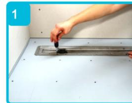
Remove the screws that secure the clamping ring to the main channel. Lift out the clamping ring and screws. Set aside.
