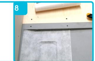
Lift up the tanking mat and gently removing the backing tape approx 300mm at a time, apply pressure to the mat and stick down. Fold the mat into the tray the other end and trim with a sharp knife.
