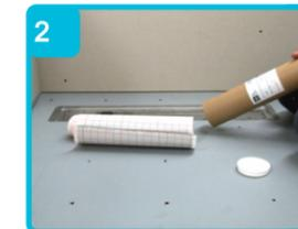
Remove the roll of tanking mat and lay over the drain. With the mat laid flat, peel the backing tape from one corner then back 150mm. Place the edge of the tanking mat against the inside edge of the tray and centrally over the channel. Apply enough pressure for the mat to adhere to the tray.
