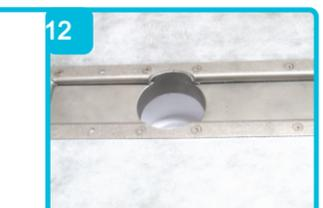
Position the clamping ring into the main channel and push down. Screw the clamping ring to the main channel through the tanking mat. With a sharp knife cut along the inside of the clamping ring and remove the excess tanking mat. Remove and replace the rest of the floor as necessary with 22mm waterproof chipboard or 24mm WPB plywood to suit.
