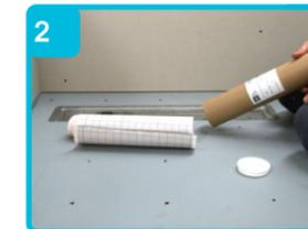
Remove the roll of tanking mat and lay over the drain. With the mat laid flat, peel the backing tape from one corner then back 150mm. Place the edge of the tanking mat against the inside edge of the tray and centrally over the channel. Apply enough pressure for the mat to adhere to the tray.
