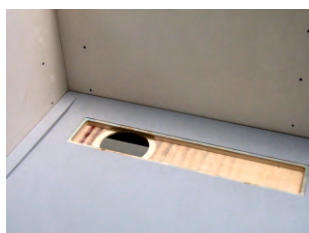
1. Lay the tray in position.
