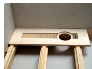
2. If the position of the waste outlet is obstructed (eg. by a joist or pipe) unscrew the waste support from the tray and turn it through 180 degree. Attach the waste support in the new position to the wall.
