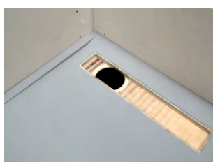
3. With the waste support attached to the tray, measure and cut off the excess material from the wall edge of the tray, to obtain a flush finish from the inside edge of the tray to the finished wall surface.
