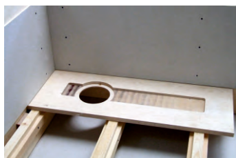
2. If the position of the waste outlet is obstructed (eg. by a joist or pipe) unscrew the waste support from the tray and turn it through 180 degree. Attach the waste support in the new position to the wall.
