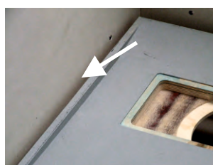
3. With the waste support attached to the tray, measure and cut off the excess material from the wall edge of the tray, to obtain a flush finish from the inside edge of the tray to the finished wall surface.
