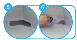
Applying OTL 028 (Internal Corner) or OTL 029 (External Corner)
