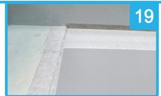
**Narrow Butyl Tanking Tape 1** Peel one side of the backing tape 150mm back from one edge. Place the end of the tanking tape against the wall and over the joint between the former and new floor, ensuring the length of the former is covered and the tape is pressed down firmly fold back the other side of the tape and remove the backing, press the tape over the edge of the former and firmly into the angle so that it overlaps the external edge of the former and the large tanking mat.
