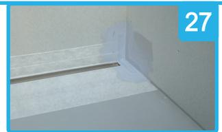
**Ensure all the Butyl Tape** is in position and pressed down firmly paying particular attention to the corners and ends. With a sharp knife cut out and remove the excess tape from the inside of the channel.
