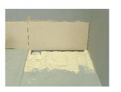
18. With the floor fully tanked and cured place the wall tile into the ledge on the channel and check for level.
