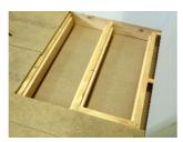
5. Secure 50mm x 25mm softwood battens 18mm below the top of the joists using 50mm x No 8 countersunk woodscrews@ 150mm centres. ready to receive 18mm WPB Plywood panels laid between the joists.
