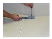
23. Place the supplied Tiling Plate Extraction Tool into the slot, turn at right angles to lift the tiling plate up to gain access to the trap.
