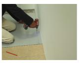
8. Secure the waste support and plywood to the joists and floor as described in instruction No 6, lay the former into position and gently lift up the channel enough to slide the former underneath the channel and in position. With the former in position secure the channel to the former and then to the wall. Secure the former to the joists and plywood using 50mm x No 8 countersunk woodscrews @ 225 centres.
