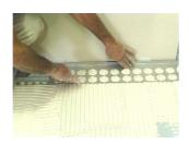
19. Place the two 8mm spacers against the wall tile. Apply a bed of tile adhesive to the floor, bed down the tiling frame into position against the spacers using a backward and forward motion.
