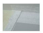
13. Peel both sides of the backing tape 150mm back from one end of the narrow tanking tape. Place the end of the tanking tape against the vertical internal corner of the drain. With the edge of the tape in line with the top of the channel work towards the opposite end of the channel. Hold the tape at 90 degrees, with a pencil mark the point where the tape meets the top of the former, cut to this point, allowing the tape to continue beyond the edge of the former and on to the wall and floor.
