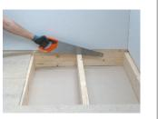
4. Place the former in position so the edge of the former is level with the surface of the wall (A). Mark out the position for the channel on the joists. Remove the former and notch out the joists to a depth of 22mm to allow for the channel.
