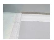
12. Peel one side of the backing tape 150mm back from one edge from the narrow Butyl Tanking Tape. Place the end of the tanking tape against the wall and over the join between the former and new floor, ensuring the length of the former is covered and the tape is pressed down firmly fold back the other side of the tape and remove the backing, press the tape over the edge of the former and firmly into the angle so that it overlaps the external edge of the former and the large tanking mat.
