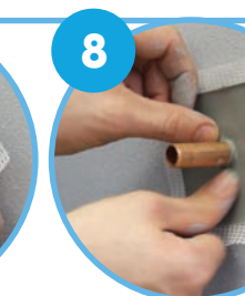
Apply OTL 026 Pipe Sleeve
