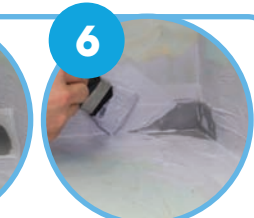
Applying OTL 028 (Internal Corner) or OTL 029 (External Corner)
