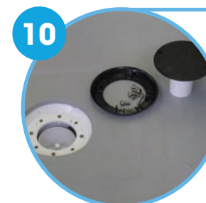
Undo the screws to the top of the trap and clamping ring
