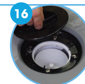
Insert the trap protector. Replace with cover when the job is complete
